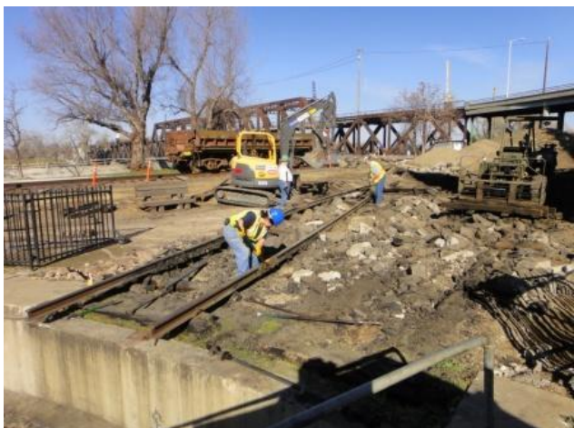
The MOW Team rips out the old tracks, January, 2012
