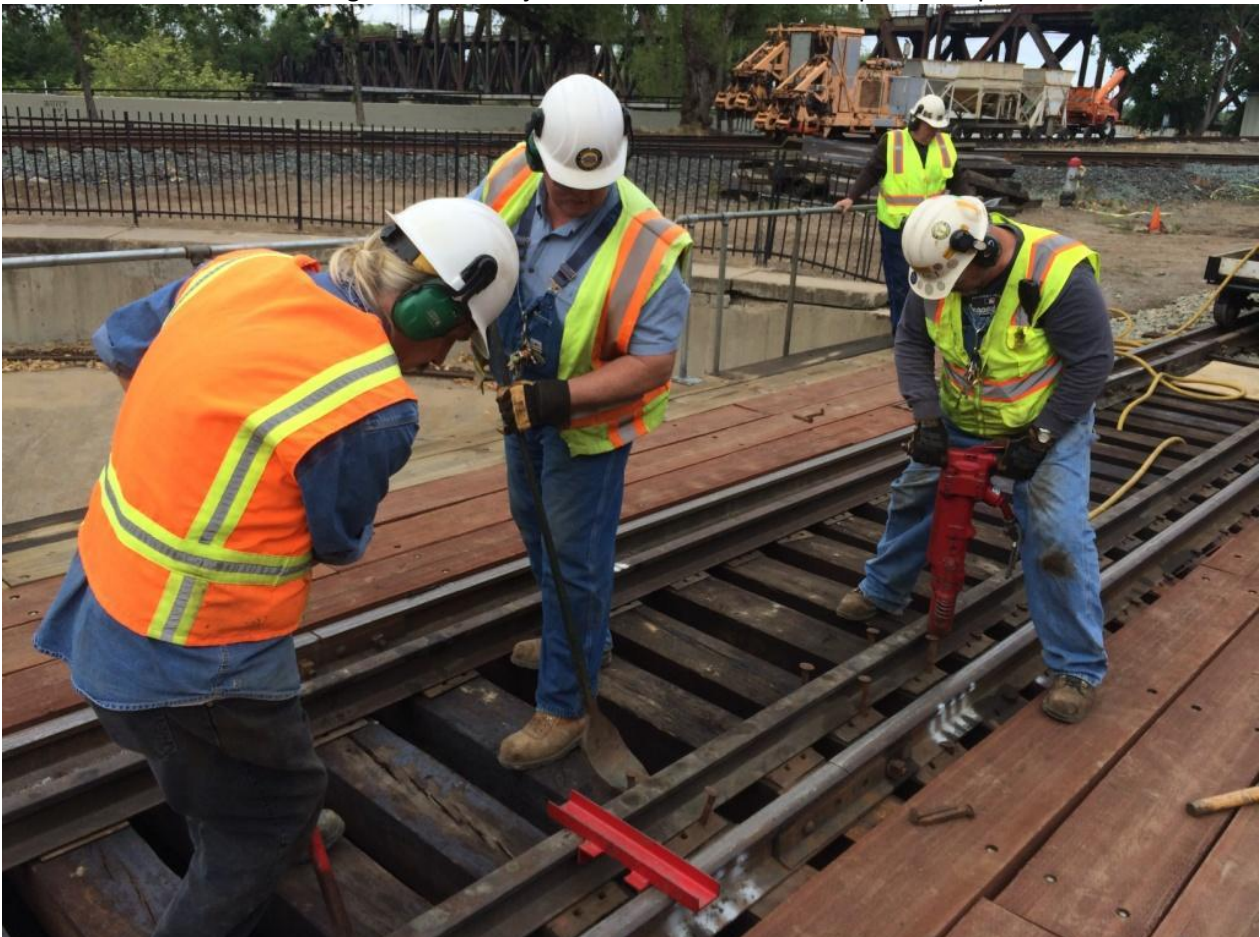
Fred and Chris shove the rail into gauge while Mike F. spikes with the pneumatic spiker
