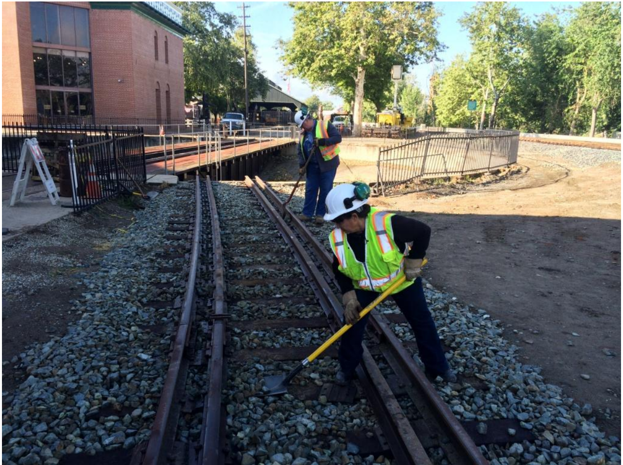
Pam and Chris smooth and straighten the ballast on the Whisker Track prior to completing the gauging operation
