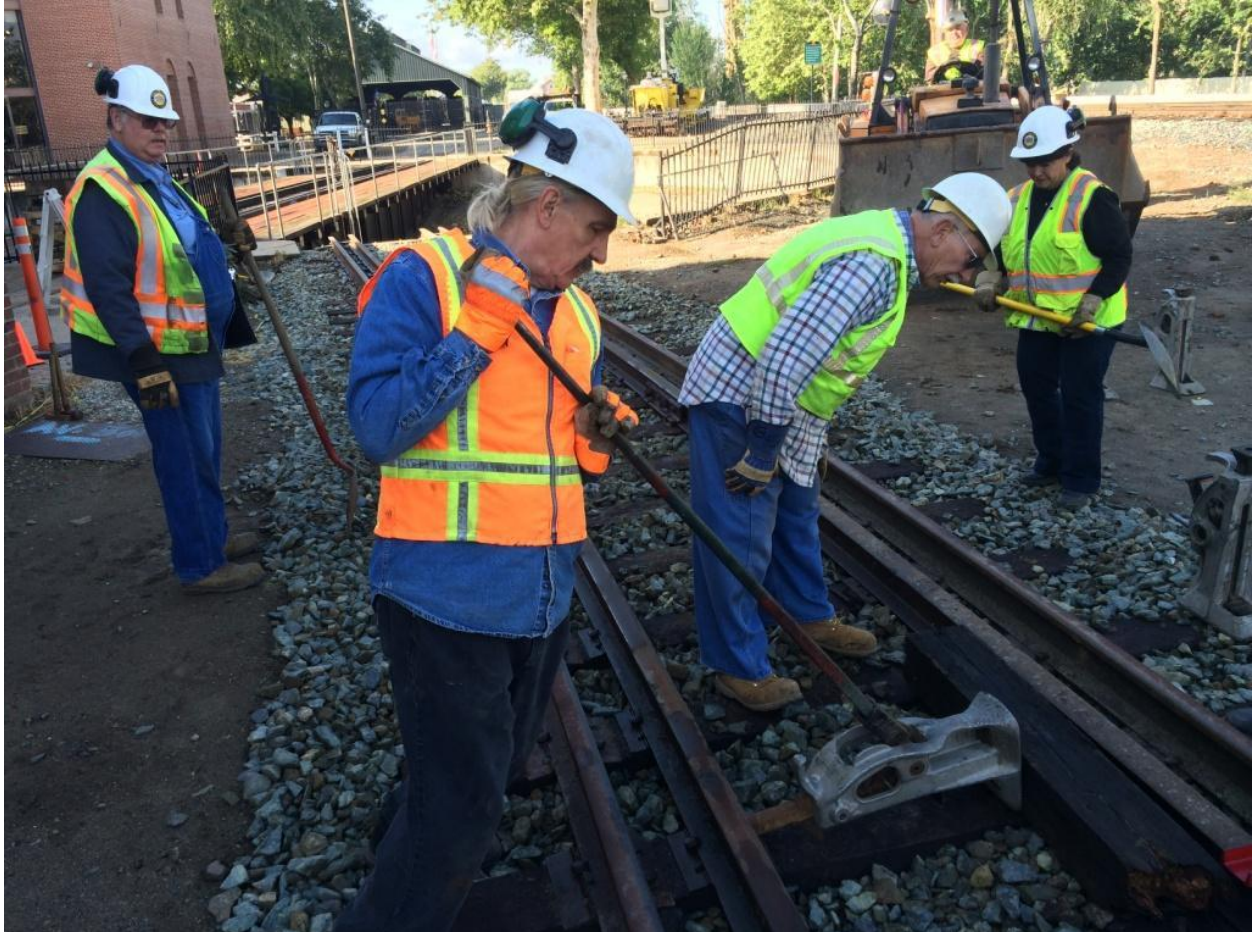
Fred and Clem use a track-jack to adjust the gauge of the narrow-gauge track
